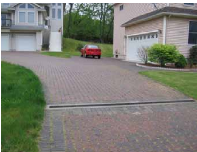
Figure 11. This shared driveway in Jordan Cove, CT helps to reduce impervious cover and is also constructed using permeable materials.
