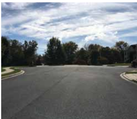
Figure 2. This cul-de-sac with a 50-foot radius creates a large bulb of rarely-used impervious cover.
